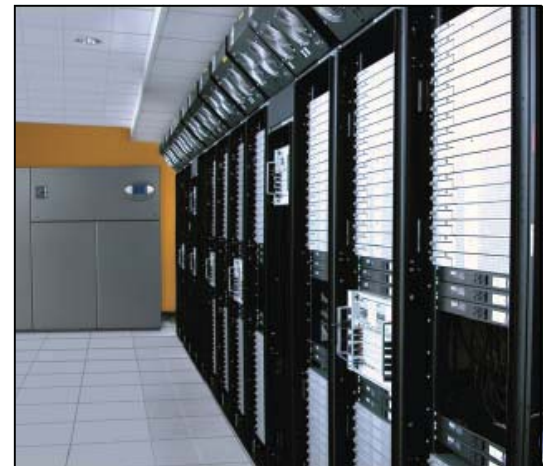
Electronic equipment puts off a dry heat, requiring more sensible cooling capacity
