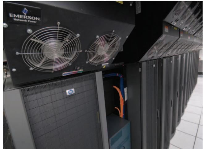
***"I was impressed by the flexibility of the different Liebert XD cooling modules. I didn't want anything touching the top of my racks that could interfere with future reconfiguration, so we suspended Liebert XDV cooling modules from the ceiling, which left clearance above the racks."***
