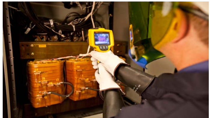
Early detection of hot spots will increase data center availability
